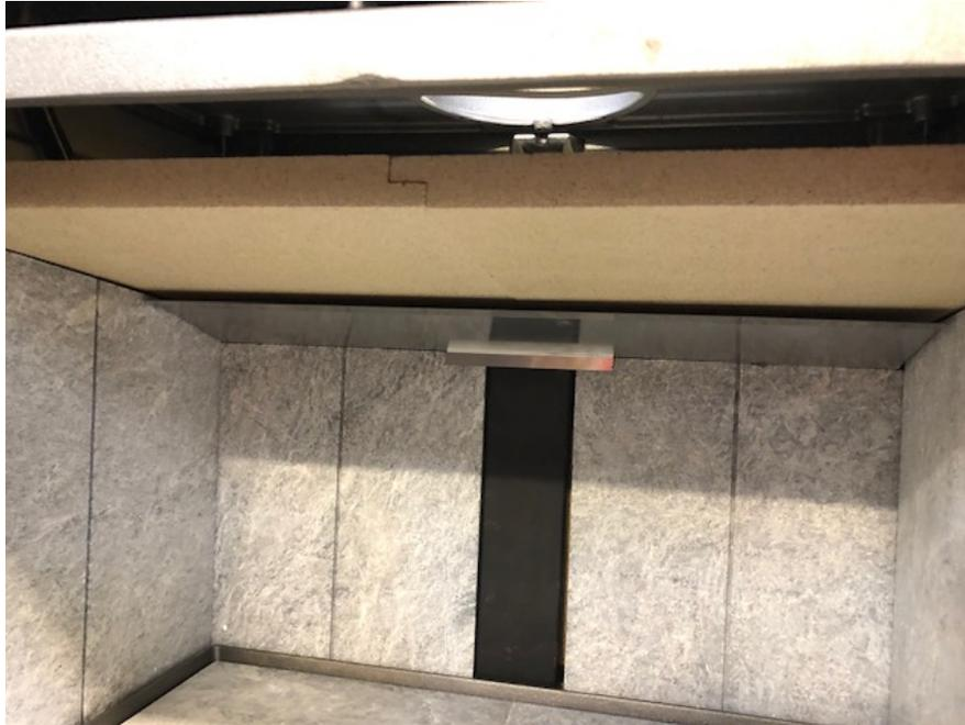
**Photo 7. Vermiculite baffles installed.**
