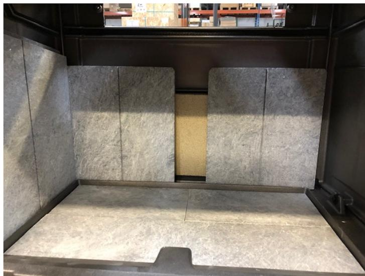
**Photo 3. Right rear refractory stone installed.**
